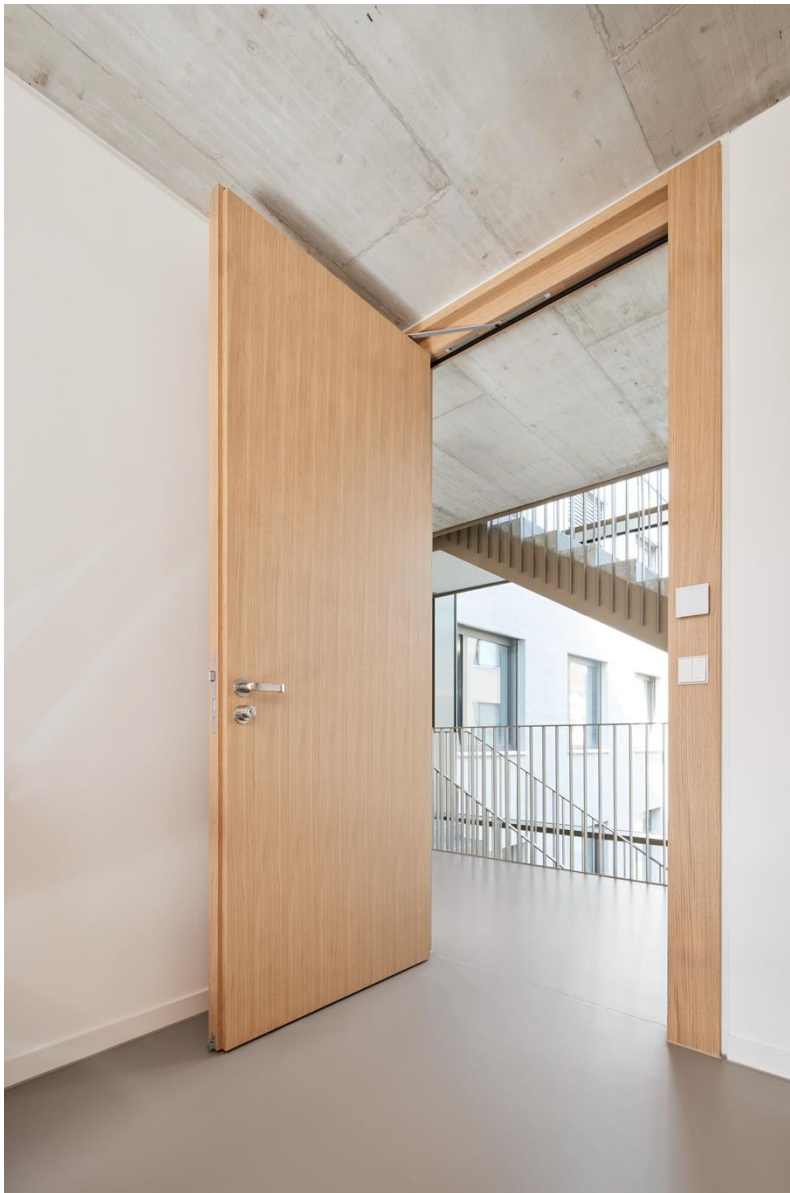
Image 12: Integrated switch boxes within the door frame.
