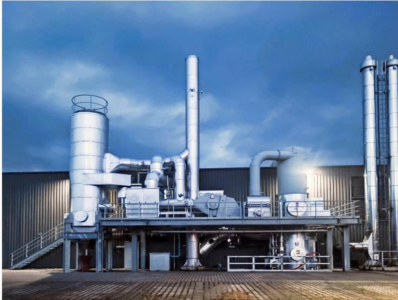
Image 5: Since summer 2021, a flue gas cleaning system at the Ampfing site has been filtering the flue gases produced by the in-house test furnace. All that remains is pure and ecologically harmless water vapour.
